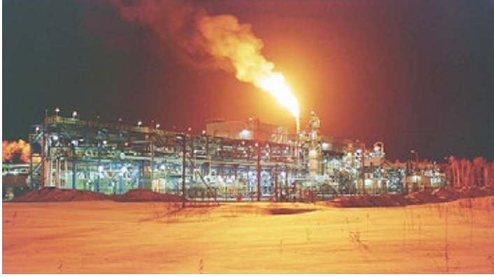
Source: Luginetsky Gas Compressor Station Strezhevoy, Western Siberia, Russia
