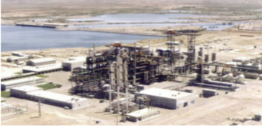
Arroyito Heavy Water Production Plant, Argentina
